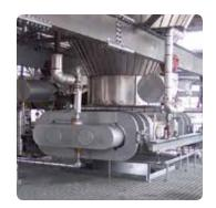
DeltaValve's bottom unheading valves are the lightest, most compact, fully automated unheading valves in the industry. The small footprint of this bottom unheading valve makes it ideal for both space constrained retrofit installations as well as new construction.
