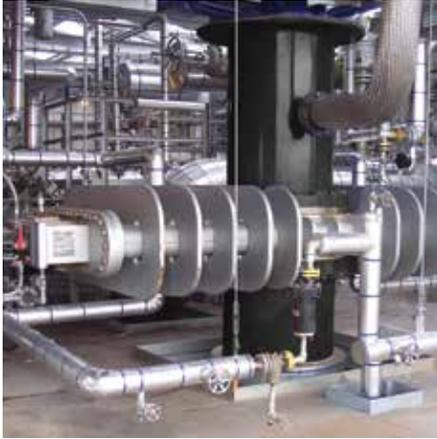
The DeltaValve top unheading valve is available in 24", 30", and 36" sizes. It is a completely enclosed system permanently connected to the top flange of a coke drum. With this valve, top drum unheading can be safely accomplished with the push of a single button from a remote location, allowing operators to be removed from the cutting deck and protecting them from potential coke drum eruptions and top head blowouts.
